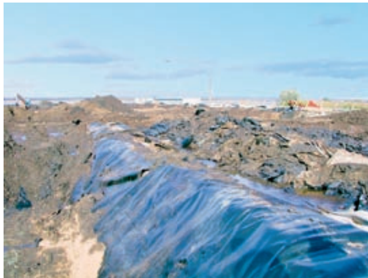
19,000 tonnes of spilled oil produced more than 300,000 tonnes of waste.
