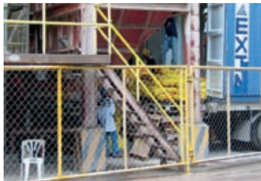
The semi-automatic co-processing facility for solid waste
